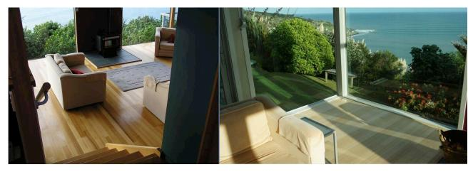
The photo on the left shows a floor with an aged oil-modified urethane and to the right a water based polyurethane on the same floor after about a year's service. It is important to note that the sealer used will also significantly influence colour as a floor ages.
