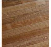
Grain discolouration – water based polyurethane
