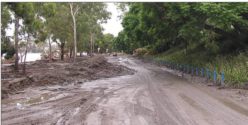
Mud and silt from the Brisbane River in 2011. The water rose to height exceeding the embankment to the right and inundated businesses and apartments.
