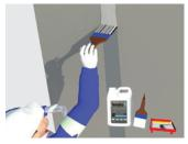
1. Apply RHINOZ Primer Bonding along the rebate joint. Leave it to dry for 10-15 minutes, or until the primer bonding becomes a clear colour.
