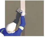
1. Apply RHINOZ Acrylic Skim on top of the Hybrid FX-55 at a thickness of <500 microns.
