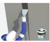
3. Apply RHINOZ Hybrid FX-55 to fully populate the rebate width and depth. Additional coats of Hybrid FX-55 are recommended to ensure the surface is left smooth and flush.
