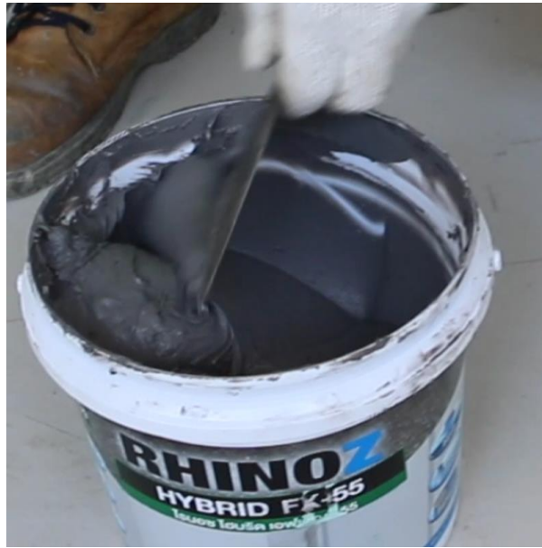
Mixing complete with homogenous colour and product from outer edge of pales mixed in.
