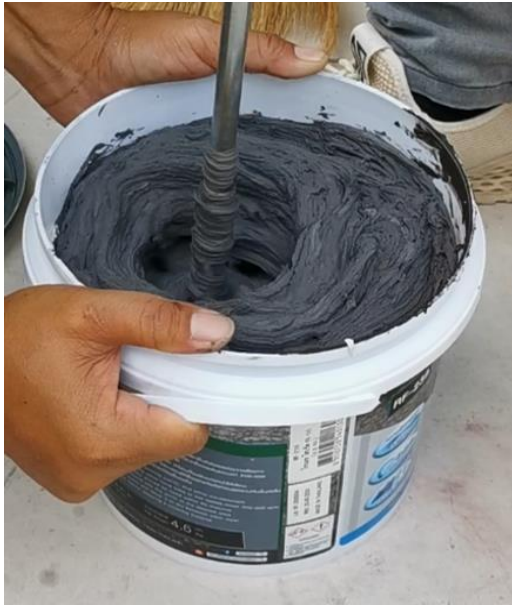
Mixing progressing to completion.
