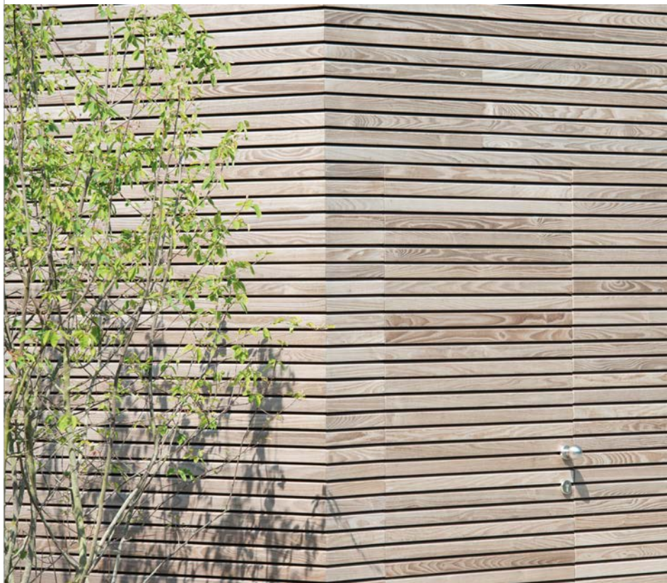
Cut the boards to a 45-degree angle.
